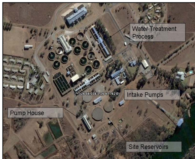
Overhead View of Midvaal Water Company site facilities
